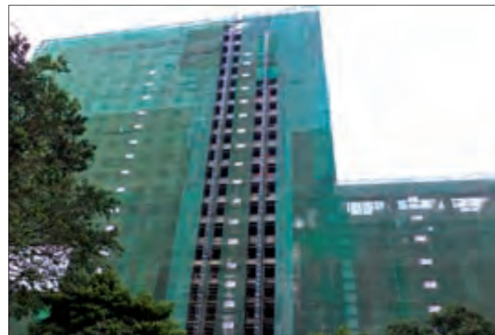
Unfinished Yangon high-rise buildings seen.
