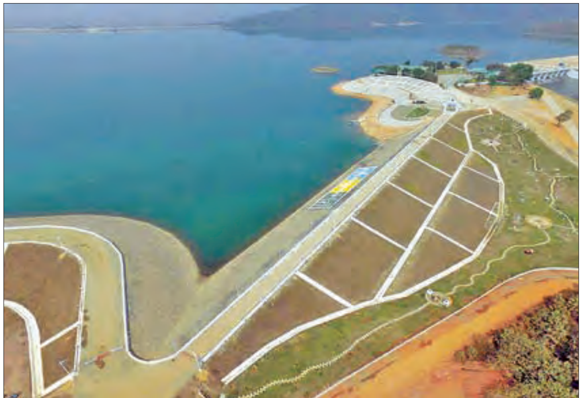
Aerial view of Yazagyo Dam. PHOTO: MNA
