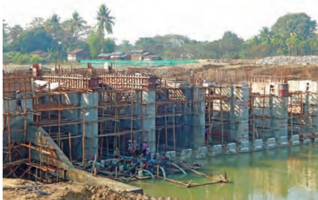
Mezali sluice gate being seen under construction. PHOTO: SOE WIN (MLA)
