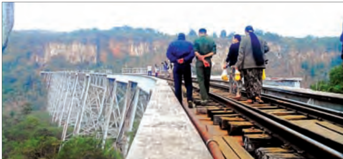
Gokhteik Viaduct. PHOTO: KO NAY
