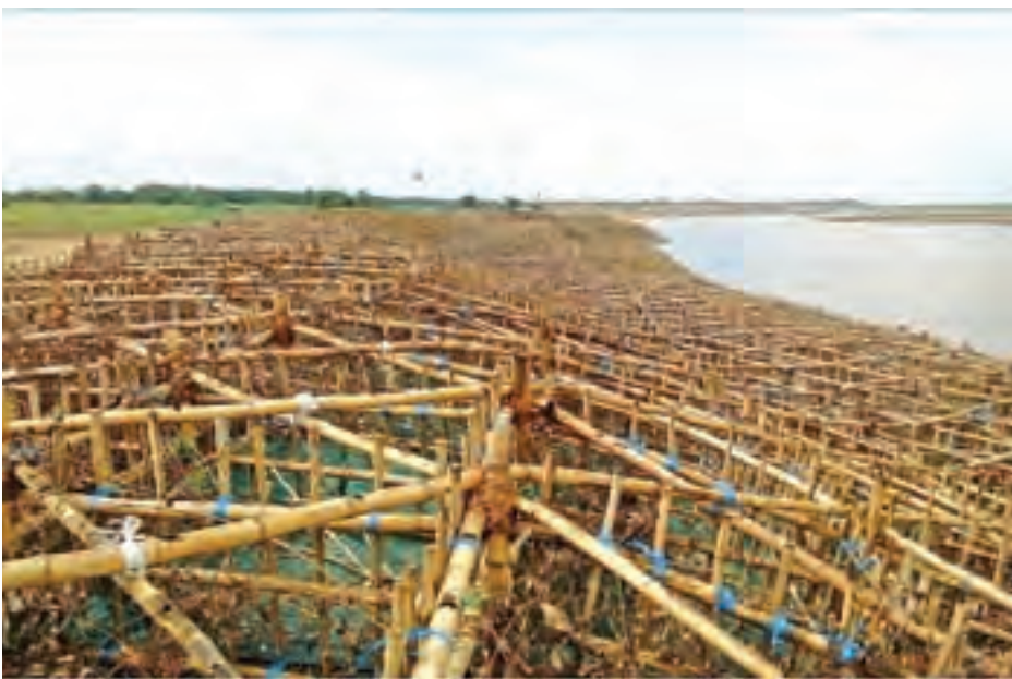
Local authorities and residents volunteered to reinforce parts of the Nyaungdon embankment as erosion destroyed parts of them during the last monsoon.
