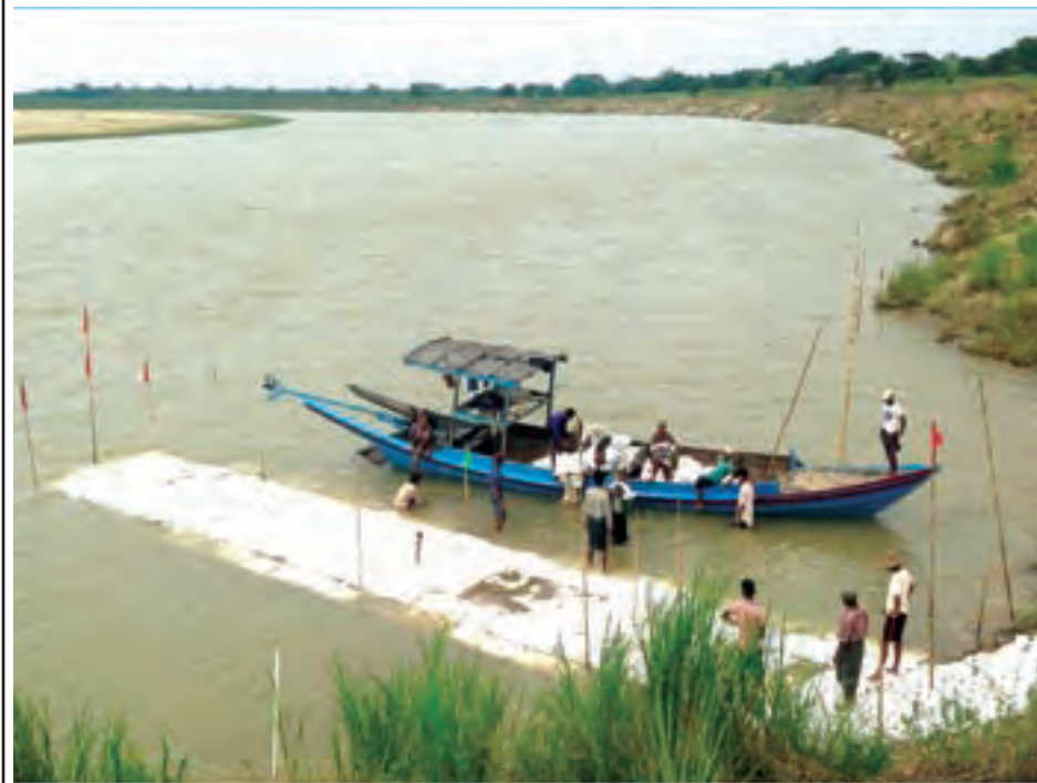
Local people and authorities are taking preventive measures laying sand bags and making bamboo lattice to manage river system and to prevent erosion in Ayeyawady Region.
