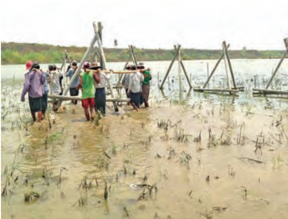
Local people and authorities are taking preventive measures laying sand bags and making bamboo lattice to manage river system and to prevent erosion in Ayeyawady Region.
