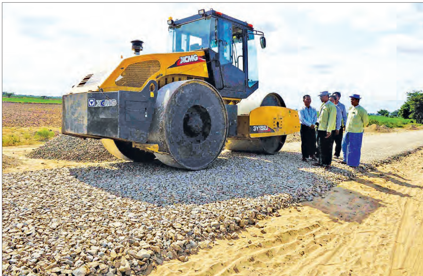
Local authorities inspect progress of Talok-Simeegon asphalt road in Myingyan Township.—ZAW MIN NAING
