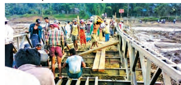
Local people participate in repairing bailey bridge on Khampat-Kanan road.—TAMU IPRD
