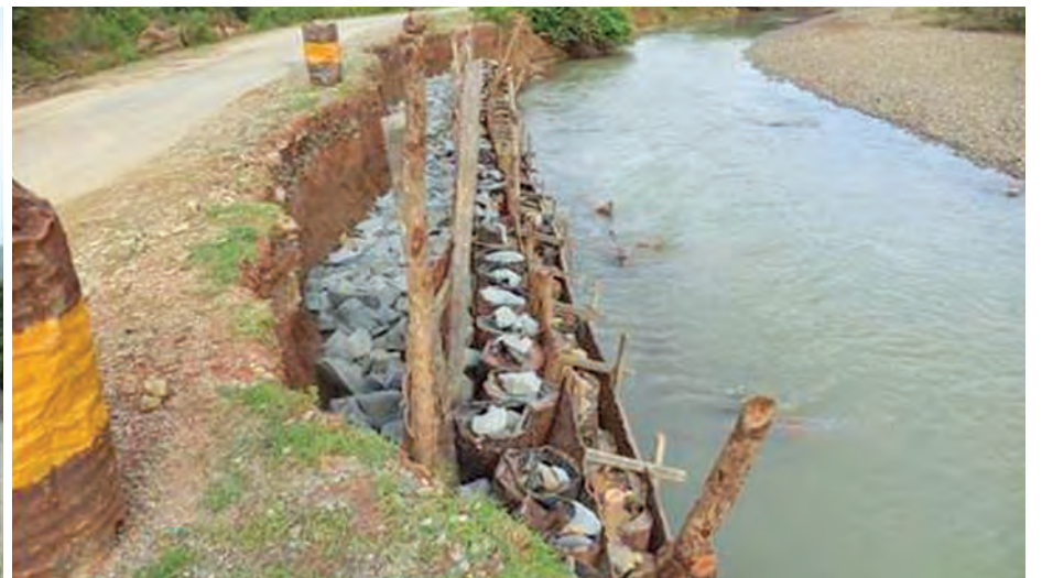
Embankment on Yangon-Sittway Road was collapsed but engineers of the Ministry of Construction has retained it by filling stones.
