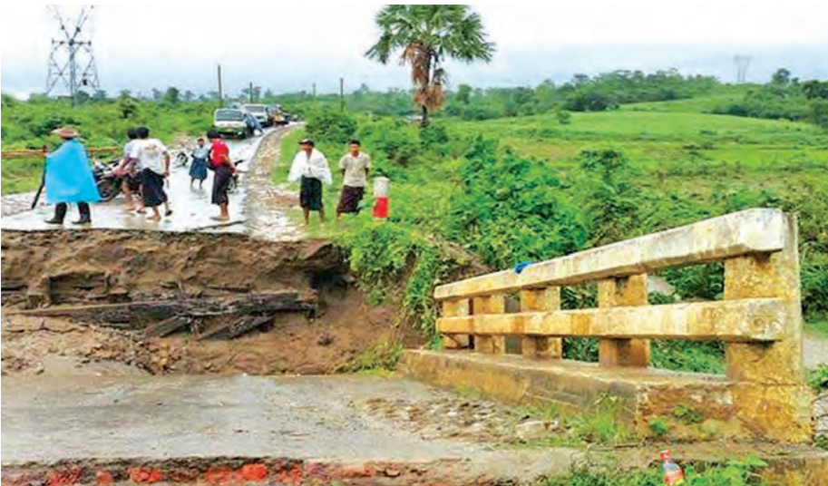
A concrete bridge on a road linking Mandalay and Myitkyina in Kachin State was damaged severely. Myanmar engineers urgently substituted the bridge with the Bailey bridge and now it is serviceable.
