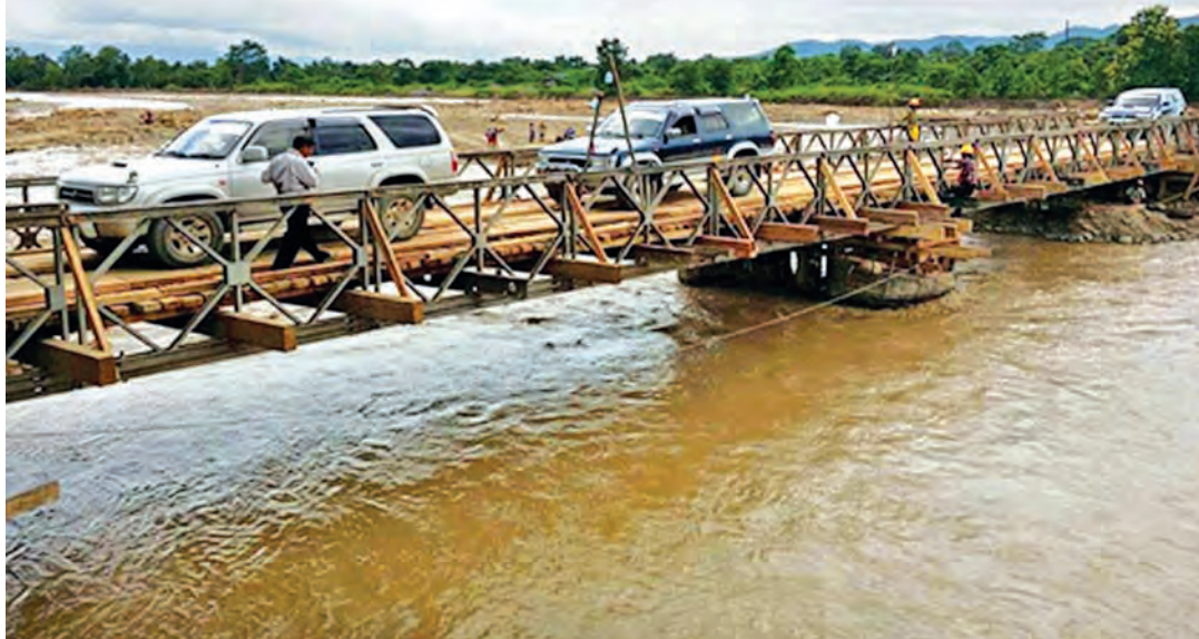
Kanan bridge on Kalewa-Kyikon-Tamu Road in Sagaing Region was destroyed by strong current. It was substituted with Bailey bridge by Ministry of Construction and now is in service for vehicles.— CONSTRUCTION
