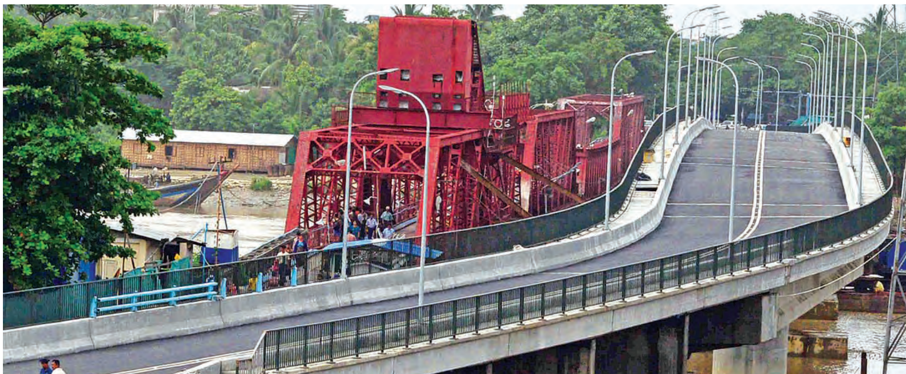
Ngamoyeik Bridge which was constructed at the cost of K 6.153 billion in Mingala Taungnyunt Township will be opened to traffic on 26 July, 2015.
