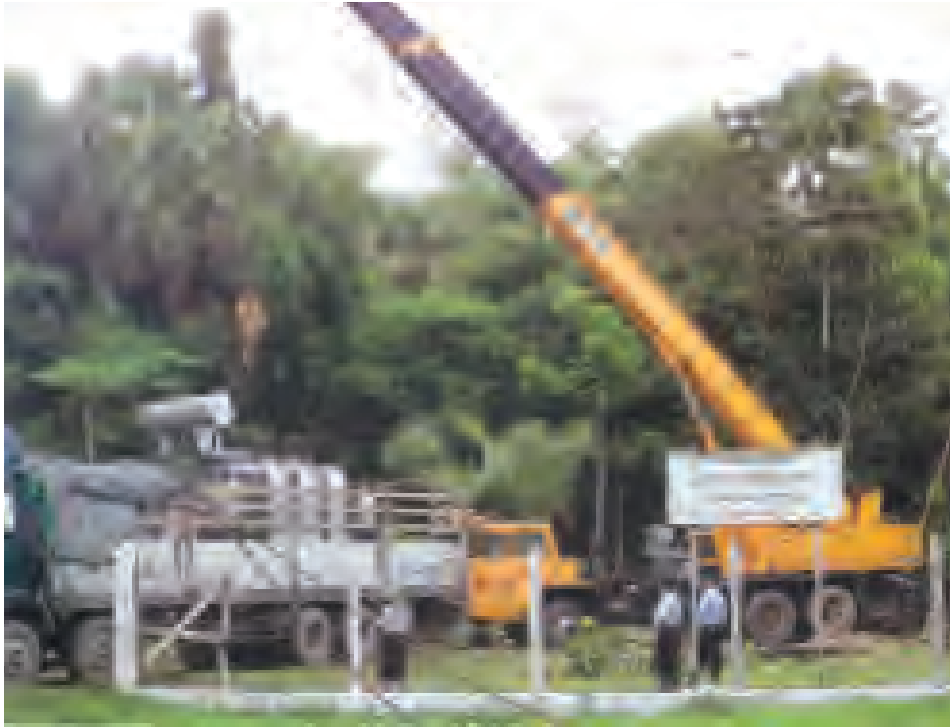
Engineers and skilled workers carry out substitution of 2500-KVA transformer in place of 1250-KVA transformer at sub-power station in Kyaunggon Township, Ayeyawady Region, on 10 June, under supervision of the Pathein District Electrical Engineer. DAVID (KYAUNG GON)
