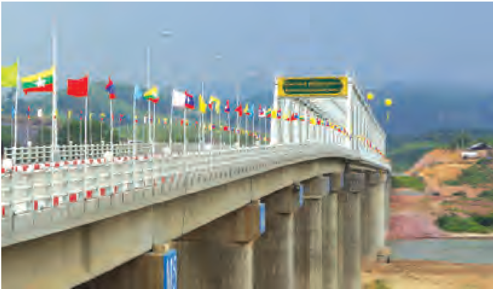
MoU on construction of Myanmar-Lao Friendship Bridge was signed in 2012 and the bridge was completed on 25 April, 2015.
