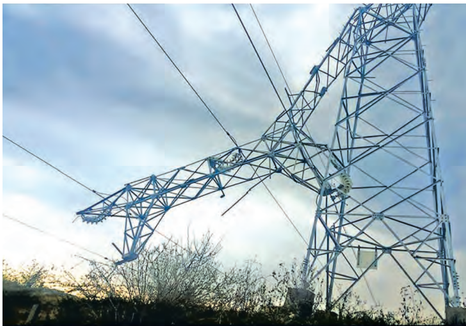
Photo shows damages of Z2 suspension tower number 144 linking Patpin and Kalaw townships near Taunggyi Township.—MNA
