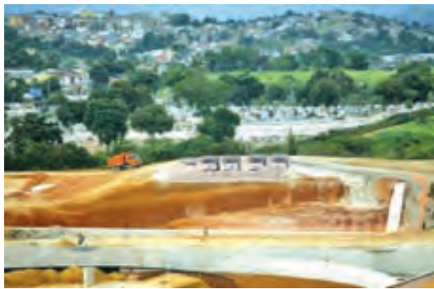
A view of construction works of the X-Park at Deodoro Sports Complex for the Rio 2016 Olympic Games, in Rio de Janeiro on 2 April, 2015.—REUTERS
