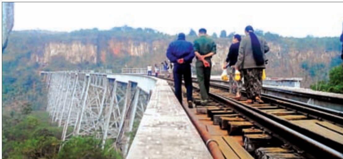
Gokhteik Viaduct. PHOTO: KO NAY
