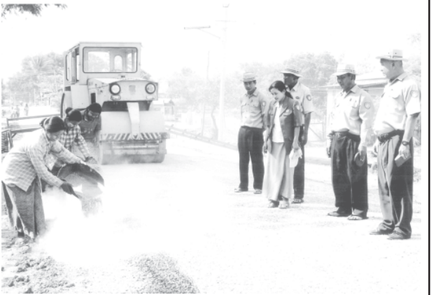
LOIKAW, KAYAH STATE : Senior Engineer of Kayah State Development Affairs Department U Min Maung and officials inspected paving of Union Road section-2 in Loikaw on 3 May, 2007. Loikaw Township Development Affairs Department is implementing the road construction projects in 2007-2008 fiscal year. LOIKAW TOWNSHIP IPRD
