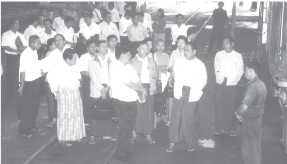
Deputy Minister looks into major repair of locomotives and production of machine parts in Insein Locomotive Shed.—RAIL TRANSPORTATION
