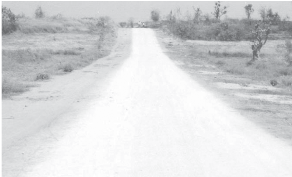
District-to-District Road No (1) in Bago Division (West) is in parallel with Yangon-Pyay Highway, about 10 miles from it. It has become a reliable transport facility for the villages at the foot of Bago Yoma mountain range.
