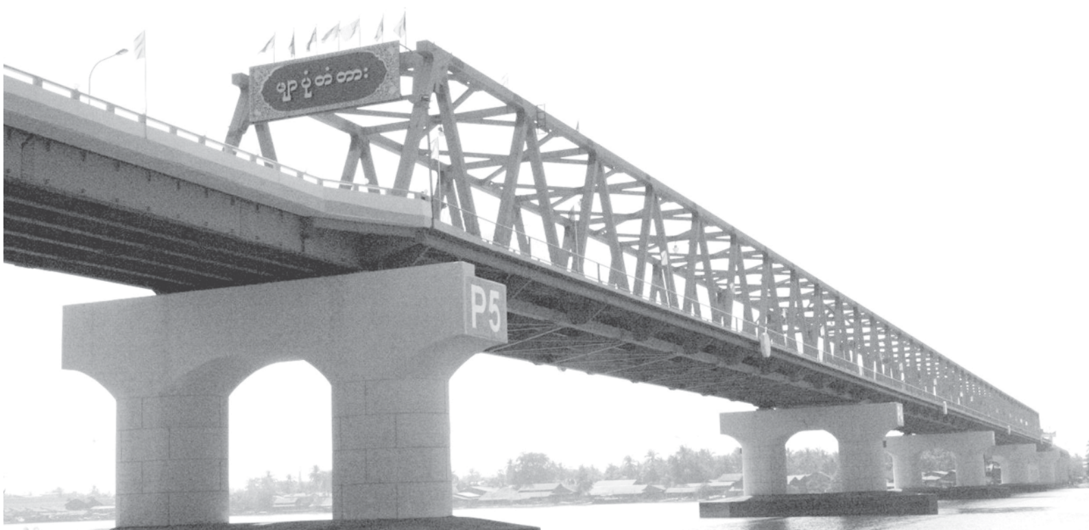
Pyapon Bridge in Pyapon Township, Ayeyawady Division. With the length of 3,933 feet, Pyapon Bridge is located on Pyapon-Dedaye-Kungyangon Road.
