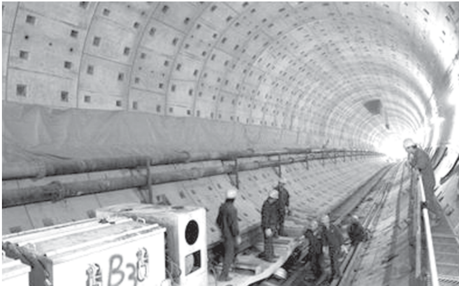
Workers inside the No 1 tunnel of the Wuhan-Yangtze River Highway Tunnel on 20 March, 2007. Construction of the Wuhan-Yangtze River Highway Tunnel has been accelerated. The tunnel lies between the Wuhan-Yangtze River Bridge and the second Yangtze River Bridge in Wuhan and will be the first to cross the Yangtze River. The tunnel is 3,630 meters long and will be open to traffic by the end of 2008. —XINHUA
