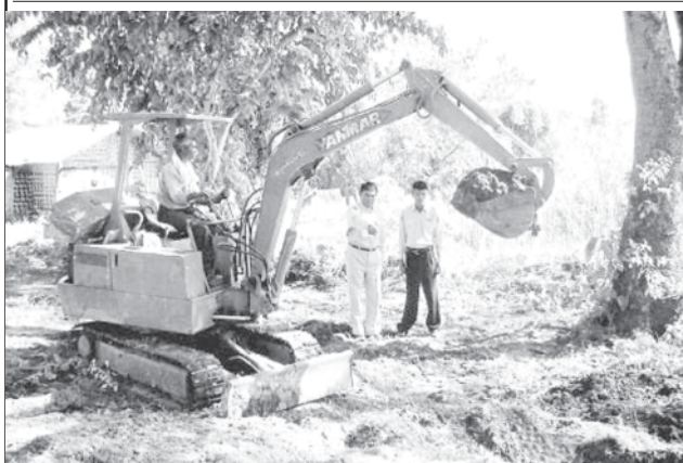
Deputy Director U Tin Win and Senior Engineer U Naing Lin of Kyaukme Township Development Affairs Committee supervised dredging of drains along Pyidaungsu Road for proper flow of water on 26 January.
