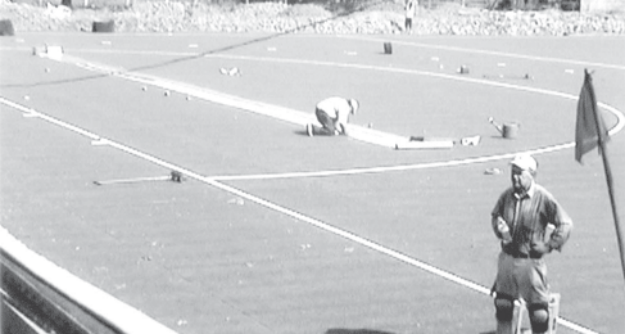
Experts of Polytan Company participate in construction of artificial turf. — MHF
