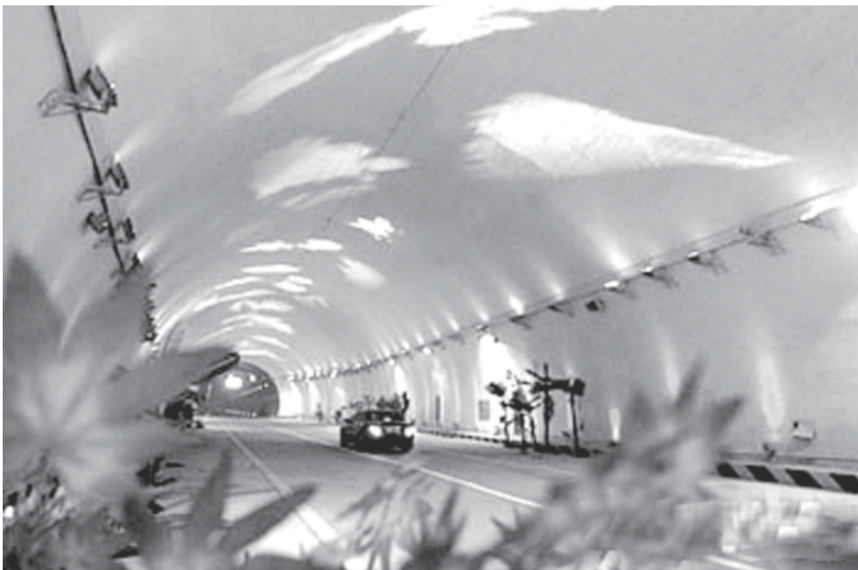
Photo taken on 17 Jan, 2007 shows the general view of the Zhongnan Mountains Tunnel in northwest China’s Shaanxi Province.—XINHUA
