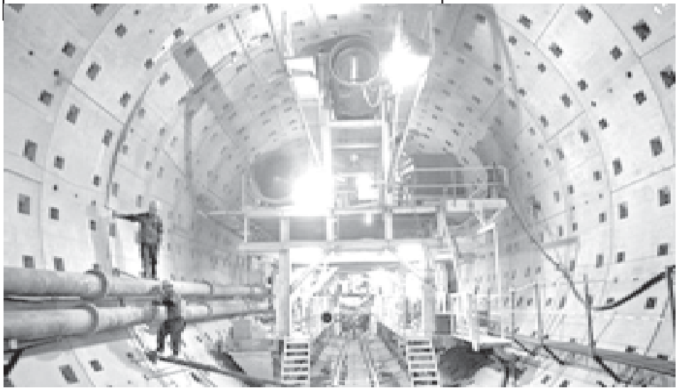
Workers work on the walls of a 3930 metres long tunnel crossing the Yangtze River in Wuhan, central China’s Hubei Province, on 7 Jan, 2007. INTERNET
