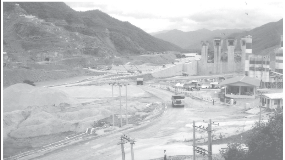
Aerial view of Yeywa Hydel Power Project site. — NO 1 EP
