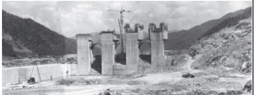
Progress in construction of Power Intake of Yeywa Hydel Power Project implemented by No-2 Construction of Hydro Electric Power Department on Myitnge river.
