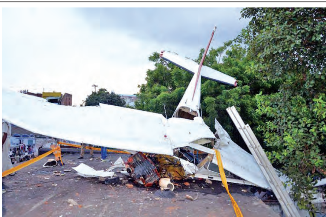
A glider aircraft is crashed on the roof of a building at Babu Purwa in Kanpur, India on 3 Sept, 2014. The pilot of the glider was seriously injured in the incident according to the report.—XINHUA
