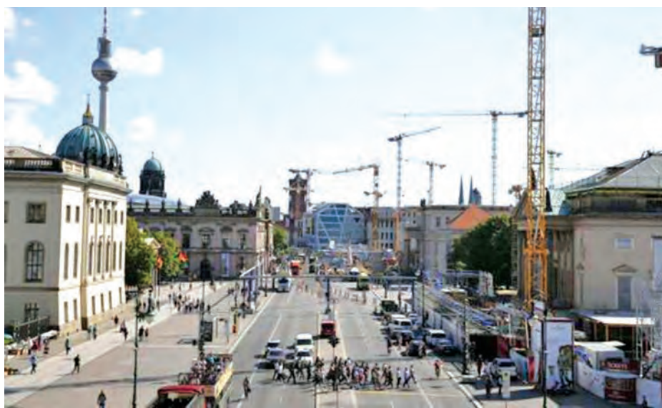
A general view shows the old city skyline at Unter den Linden street with the construction site of the Berliner Schloss (Berlin City Palace) — Humboldtforum (C) in Berlin, on 28 Aug, 2014. — REUTERS
