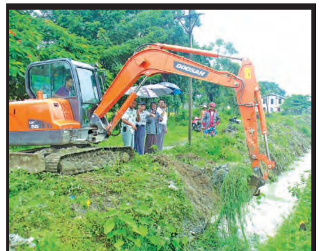
Kachin State level officials supervised dredging of 3,500 feet long, seven feet deep and six feet wide drain in Myathida Ward of Hopin in Kachin State on 1 and 2 August. TOWNSHIP IPRD
