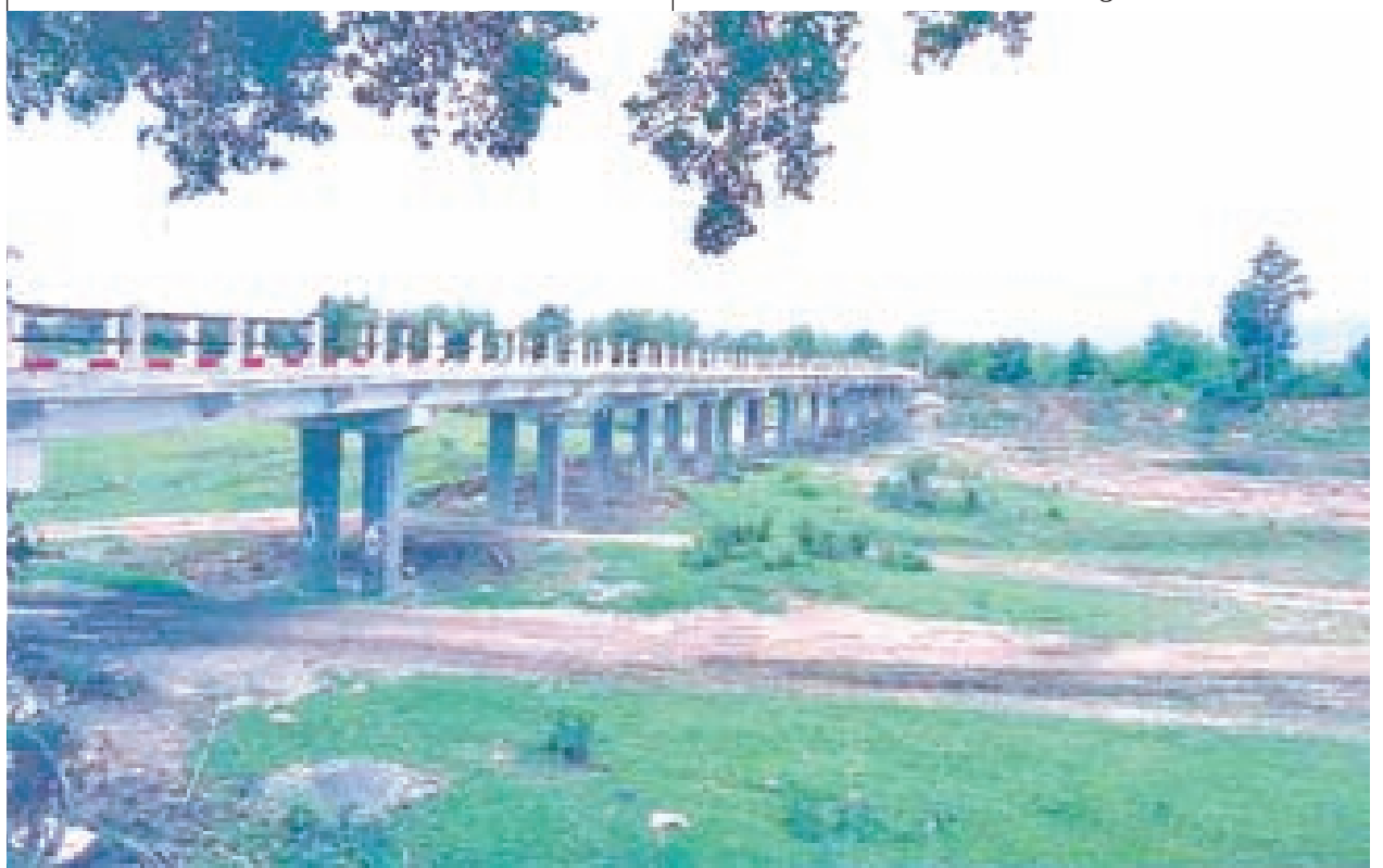
Photo shows newly-built reinforced concrete bridge across Nantyin Creek in Mohnyin Township.
