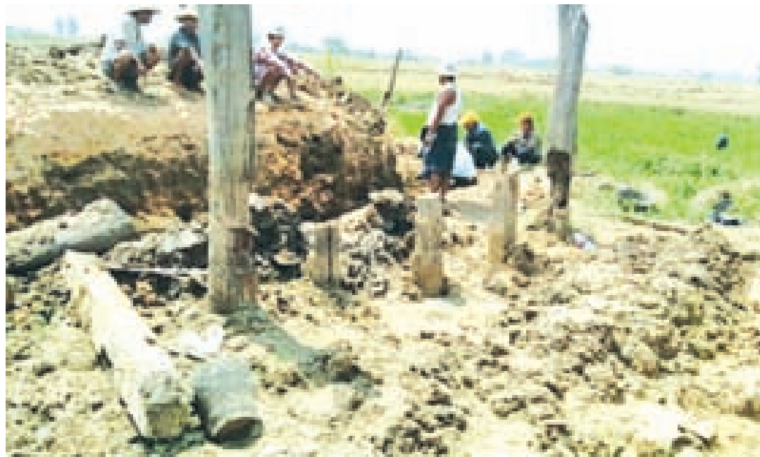
Photo shows work on construction of a bridge in Pobbathiri Township in Nay Pyi Taw Council Area. NLM-003
