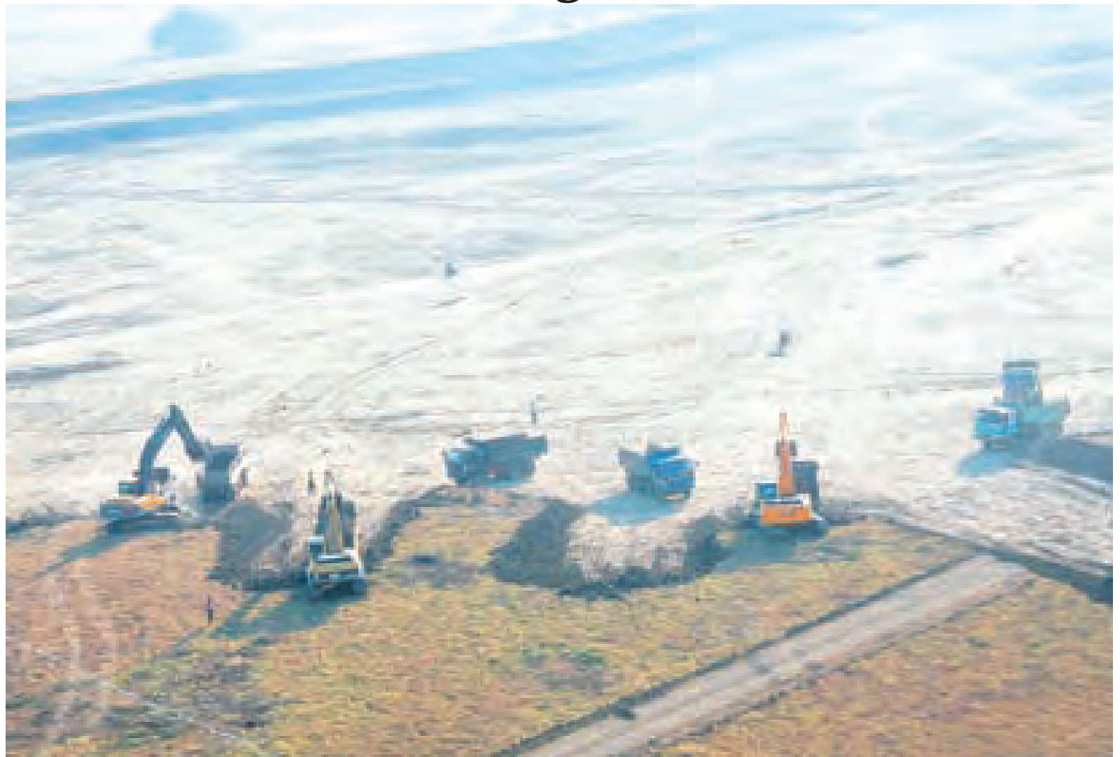
Silted Hthilaing Lake is under dredging and renovation in Wundwin Township.—MNA
