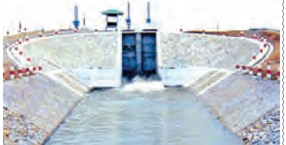
Sluice gate of left main canal at Khabaung Dam
