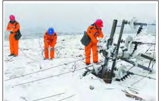
Workers of power supply company repair transmission line in Erxianyan Village of Huolongping Township in Xianfeng County, central China's Hubei Province, on 16 Feb, 2014. Due to the snowstorm in recent days, electricity grid in Enshi Tu and Miao Ethnic Autonomous Prefecture was badly damaged and employees of the power supply company have been called on to deice and repair electricity transmission lines. —XINHUA
