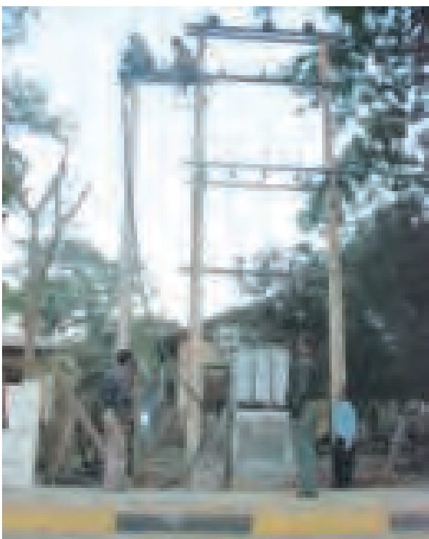
Electricians in works to move transformer to load centre of the township.
