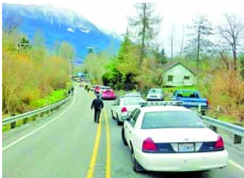
Officials and cars line the highway at the site of a large mudslide in this handout photo provided by the Washington State Police near Oso, Washington on 22 March, 2014. —REUTERS
