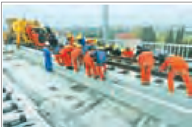
Workers lay tracks at the construction site of Hangzhou-Changsha high-speed railway in Zhuji City, east China's Zhejiang Province, on 10 Nov, 2013. The 920-kilometre high-speed railway linking Hangzhou City and Changsha City, respectively capital of Zhejiang Province and capital of Hunan Province, and designed at a top speed of 350km/h, will reduce the travel time from more than six hours to three hours after it is put into operation in 2014 as expected.—XINHUA
