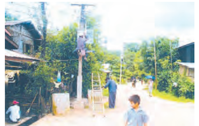
An electrician install digital electric metre.
