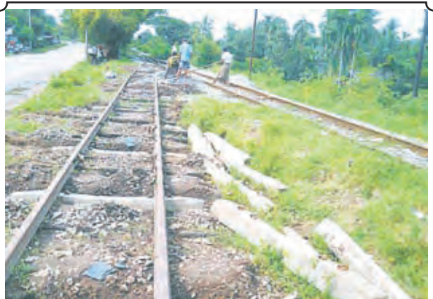
Workers of Myanmar Railways carrying out maintenance of rail tracks and substitution of new concrete sleepers along Yangon-Mawlamyine railroad at the entrance to Theinzayat Station in Kyaukse Township of Mon State on 27 August.
