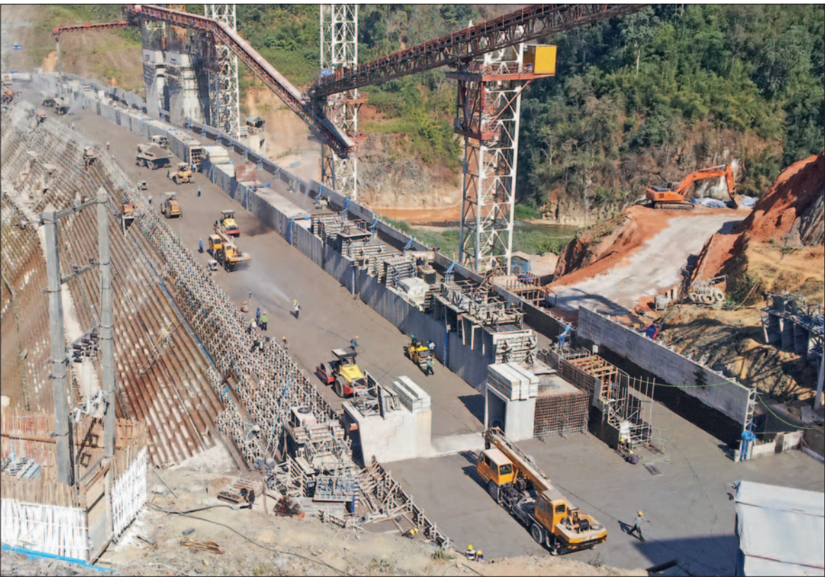
Workers build the Paunglaung dam in Shan State's Pinlaung township. Photo: Supplied/Kayan Youth Group
