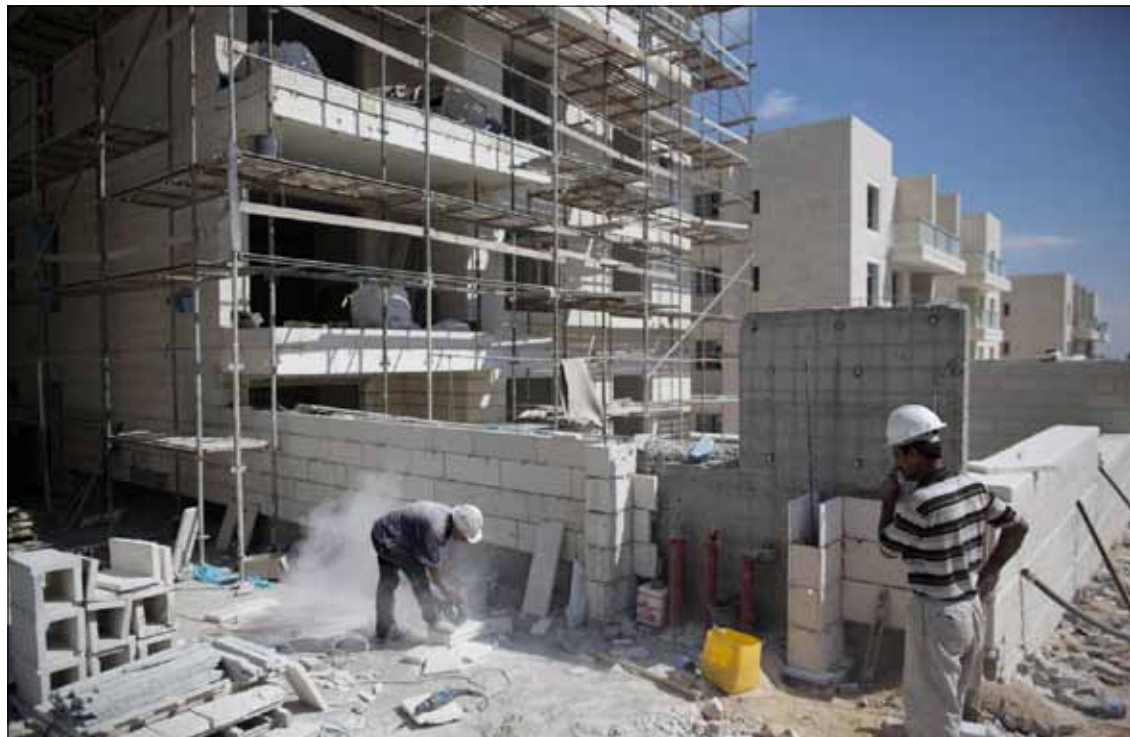
A picture shows laborers working at the construction site of a new housing project at the Jewish settlement of Gilo in east Jerusalem in April. Israel cancelled plans to build 20,000 new settler homes in the West Bank. Photo: AFP
