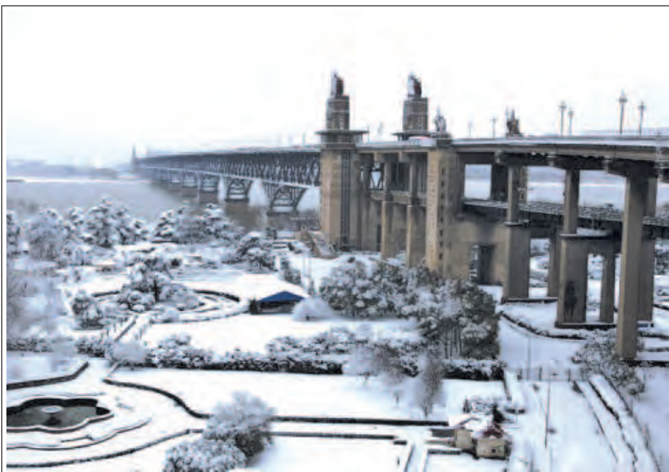
Photo taken on 19 Feb, 2013 shows the snow-covered Nanjing Yangtze River Bridge in Nanjing, capital of east China's Jiangsu Province. Many cities in eastern and central China were hit by a snowfall on 19 February.—XINHUA
