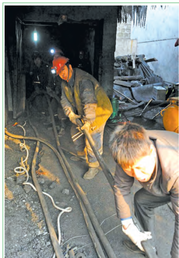
Rescuers lay the suction pipe at a coal mine in Madixiang Community of Yangquan, north China's Shanxi Province, on 19 Feb, 2013. Six people have been trapped underground since a coal mine in Yangquan City was flooded at about 4 am on Tuesday, when 12 people were conducting illegal mining operations, the local government said.—XINHUA
