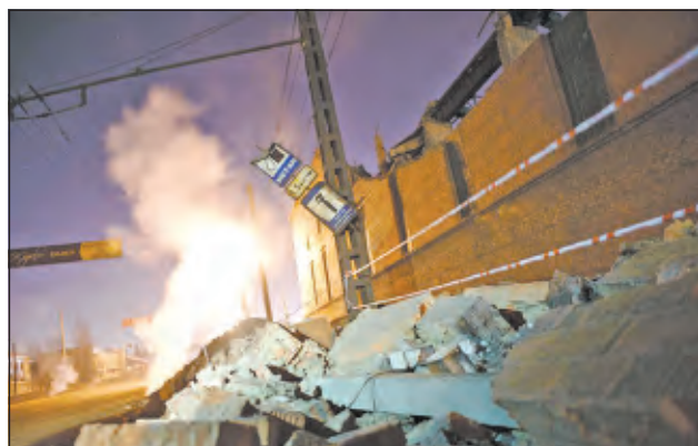
Photo taken on 16 Feb, 2013 shows a factory building damaged by the shockwave of the meteorite fall in Russia's Ural city of Chelyabinsk. Some 1,200 people have been injured and many houses damaged as a meteorite struck Russia's Urals region on Friday.—XINHUA
