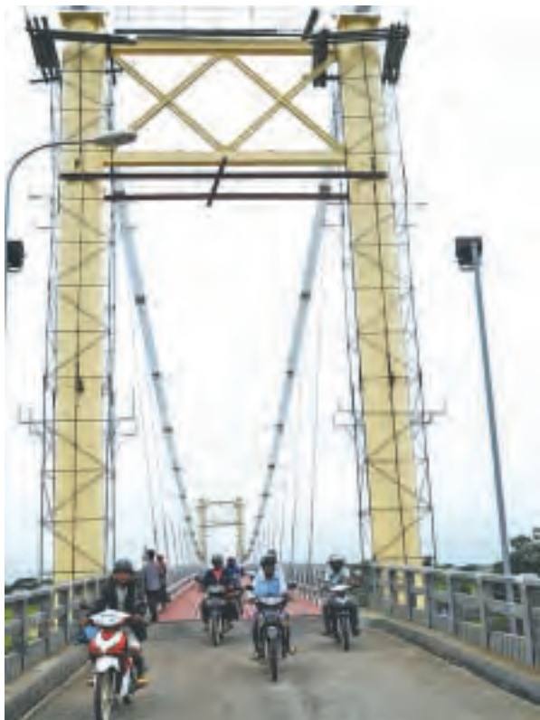
Photo shows motorbikes passing along Seikkyi-Khanaungto steel suspension bridge.
