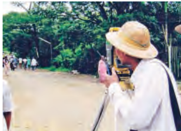
A survey team conducting preparation for topographical map.
