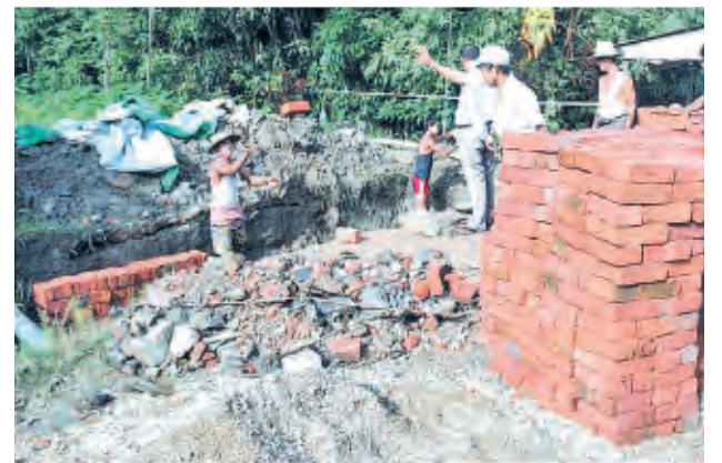
A box culvert is being built by Township Development Affairs Committee on 2 nd Aungthitsa street in Ward 3 of Pyapon for proper flow of water spending K 720,000 for prevention of flood in rainy season.—KYEMON-540
