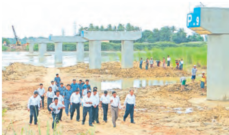
Union Minister U Kyaw Lwin visits bridge construction project.—MNA
