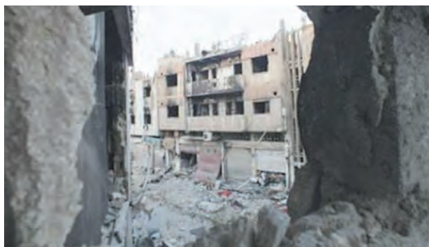
A view shows damaged buildings in the besieged area of Homs on 12 July, 2013.—REUTERS
