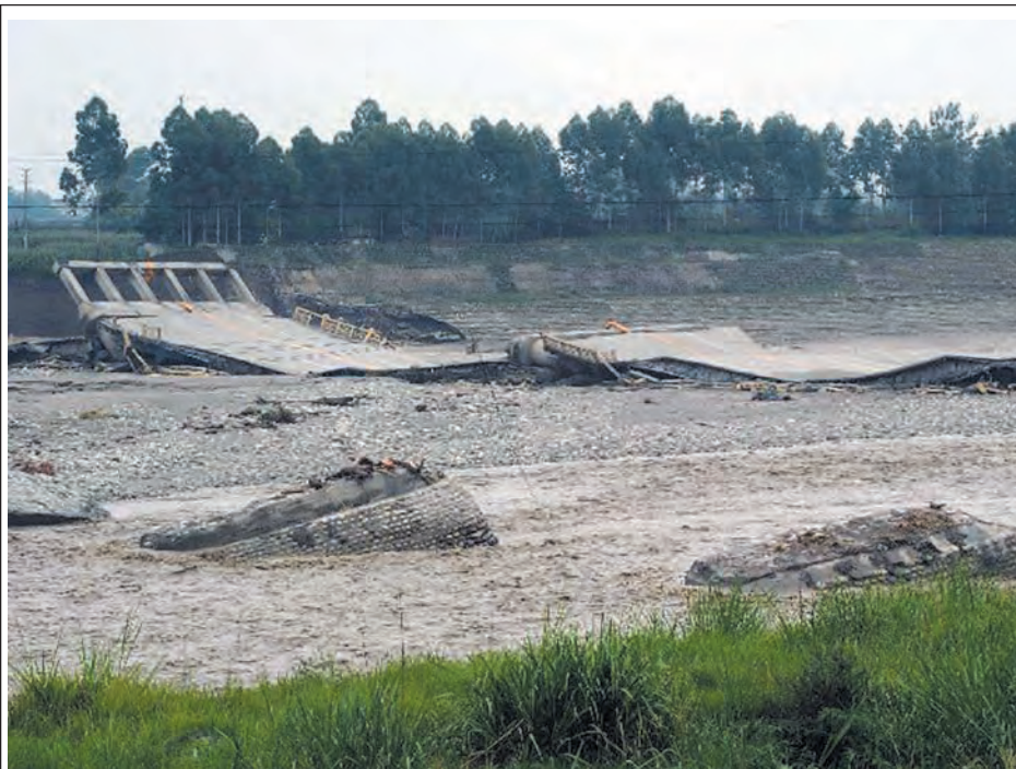
Photo taken on 11 July, 2013 shows the collapsed Chuanxi Bridge in Junyue Town of Pengzhou City, southwest China's Sichuan Province. Rainstorms battered the region these days, and the fast flow of the river water brought damages to the bridge. The damages had been found in time and the traffic had been controlled. No casualties were reported in the accident.
