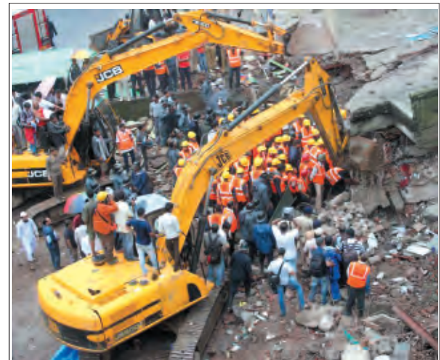
Rescuers work at the site of collapsed residential building in Thane District on the outskirts of Mumbai, India, on 21 June, 2013. Ten people were killed and several others were feared trapped under the debris of a three-storey building near Mumbai on Friday, the financial capital of India, according to local media reports.—XINHUA
