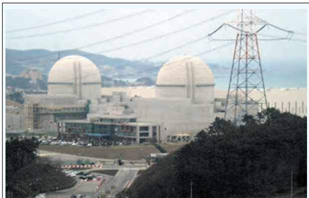
Photo taken on 5 Feb, 2013, shows dome-type Advanced Power Reactor 1400 reactors at the Kori nuclear power plant in Ulsan, South Korea. In 2009, South Korea landed a $41 billion contract to export four APR 1400 reactors to the UAE together with operational skills and nuclear fuel.—KYODO NEWS
