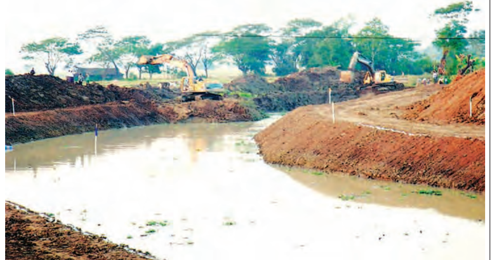
A photo shows implementation and extension works of Aung Mingalar channel in Pantanaw Township with heavy machinery.
