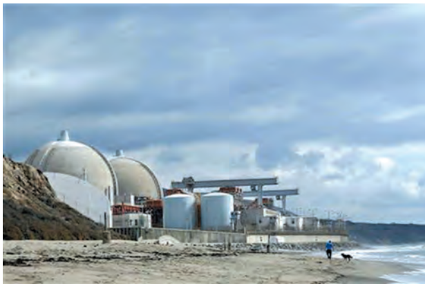
A man walks his dog next to the damaged San Onofre power plant located next to San Onofre State Park in California, in this on 8 Nov, 2012.
