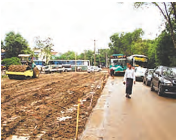
Yangon Highway Bus Terminal road under major repair.
