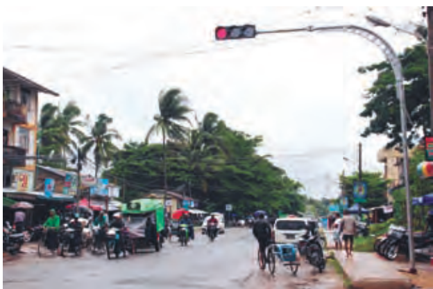
A new traffic light installed at the junction of Thanatpin road and Bandoola road in Bago.
