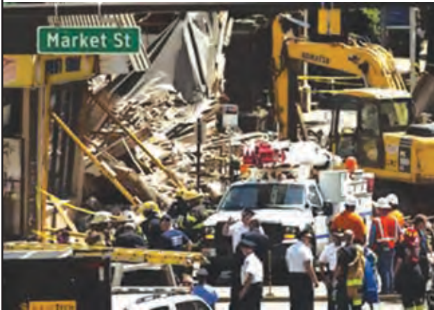
Rescue workers search through rubble following a building collapse in Philadelphia on 5 June, 2013.
