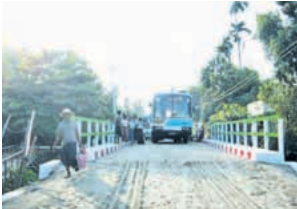
Photo shows newly-built Kyaiklat Pagoda Creek Bridge.
